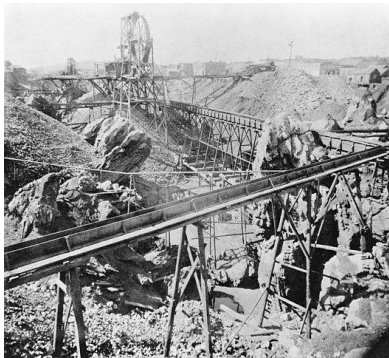
Example of ditch systems used to mine gold during the Gold Rush
